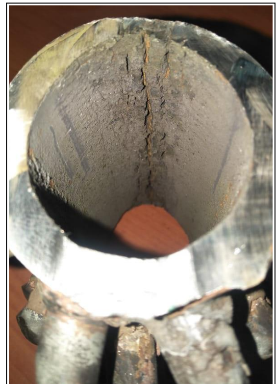
Photo 2: Inside of failed tube
