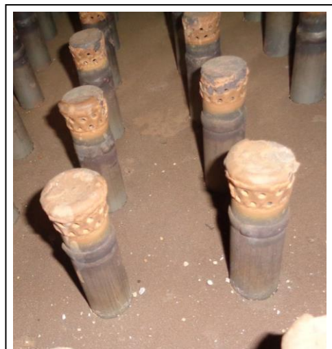
Photo 6: Plugged air nozzles
