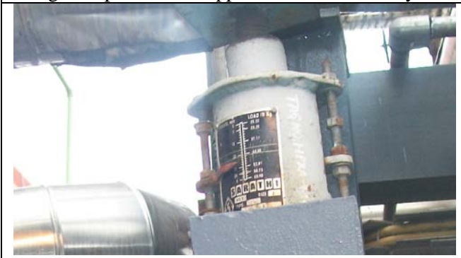
Photo 10: Pipe support partially commissioned by the commissioning team.
