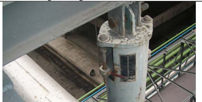
Photo 6: We can see that the spring support next to the above two supports has got overloaded.
